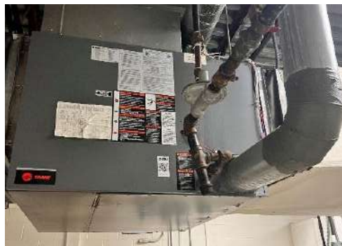
Existing Student Dining Duct Heating Coil
