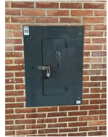
Typical Branch Circuit Panelboards in Corridor
