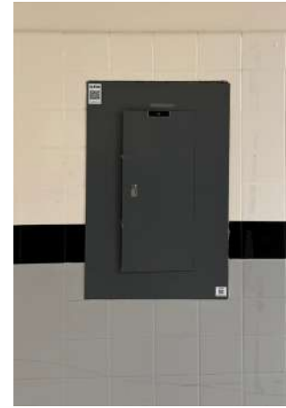
Typical Branch Circuit Panelboards in Corridor
