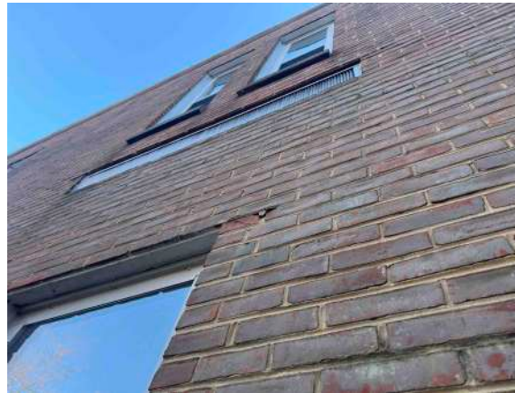
Brick Spalling
