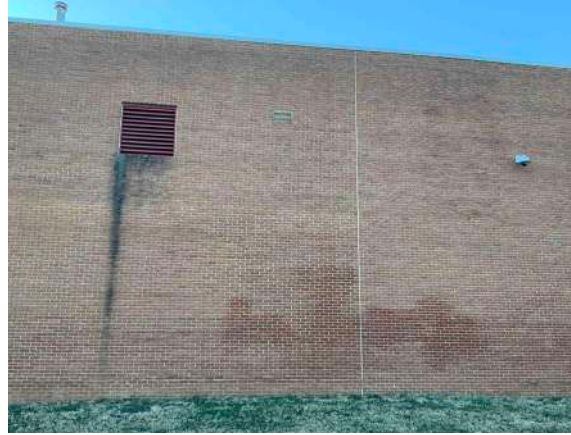
Water Infiltration Visible on Facade
