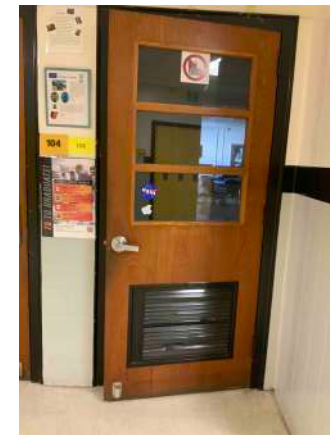
Door Louvers Transfer Sound and Smoke from Corridor
