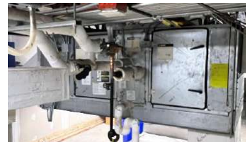
Existing AHU Serving Resource Rooms
