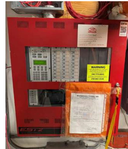
Fire Alarm Control Panel and Voice Control Panel
