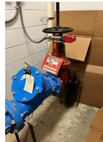
Incoming Fire Service/Backflow Preventer
