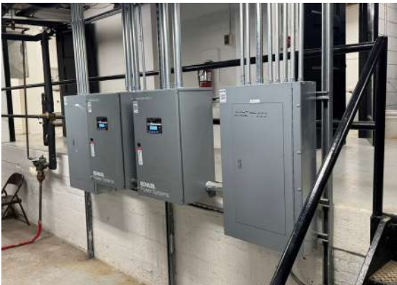
Automatic Transfer Switches
