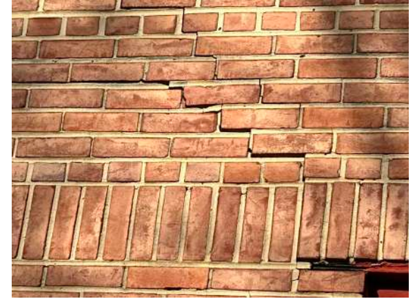
Brick Joint Degradation
