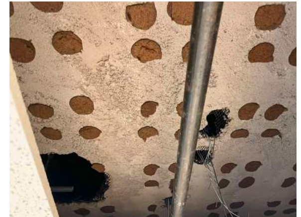
Original Plaster Ceilings Remain Above New Drop Ceiling
