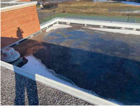
Ponding on Roof
