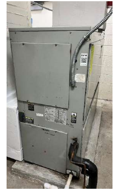
Existing Air-handling unit (AHU-3)
