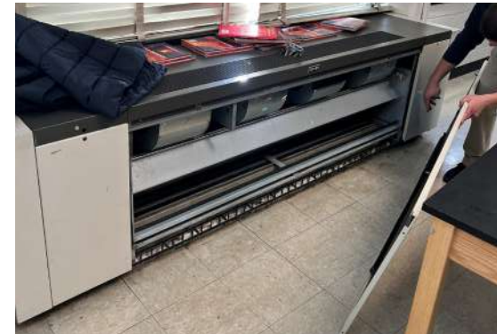
Typical Classroom Unit Ventilator
