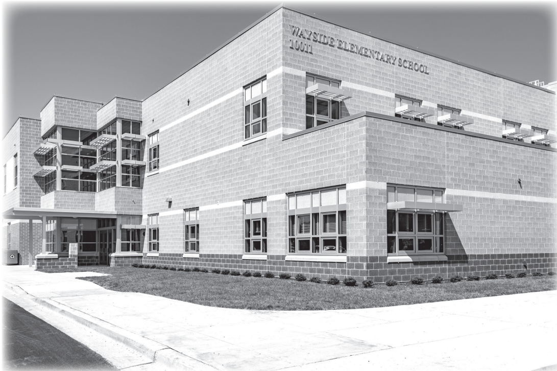
Wayside Elementary School
